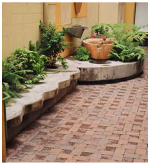
UngROUTED modular pavers promote infiltration, Berkeley
