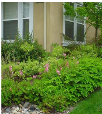
Rooftop runoff drains to bubbler in landscaped area, Fremont
