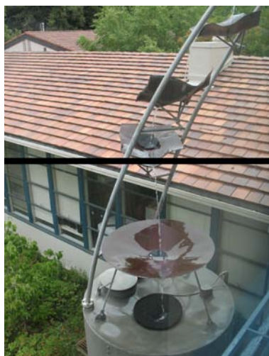
Sculpture collects and stores roof runoff at Mills College in Oakland.
