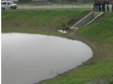
Detention pond in Pleasanton provides stormwater treatment and hydromodification management.
