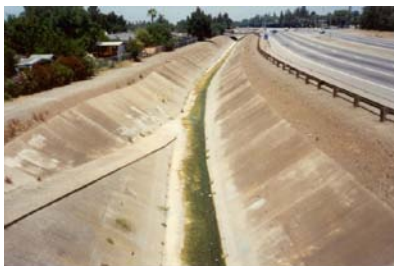
Example of an engineered channel.
