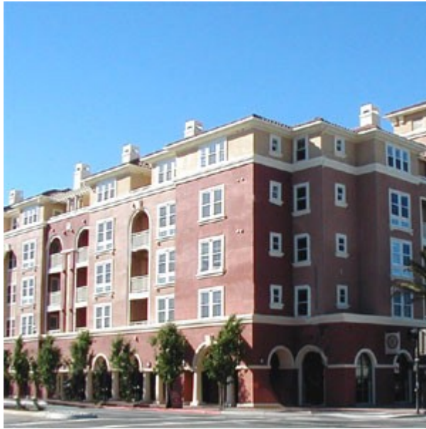
Typical Podium Building
