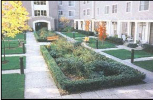
Typical Bioretention Area
