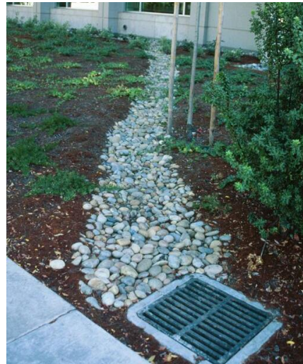
Photo 7-1. Draining roof runoff to a landscaped area is an example of hydrologic source control.
