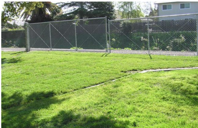
Photo 8-7. Turf block fire lane
