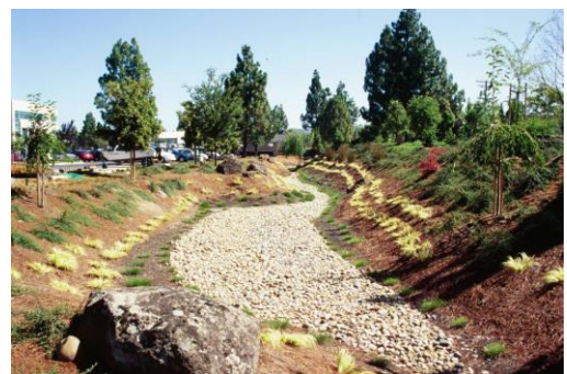
Photo 8-5. Extended Detention Basin, Palo Alto
