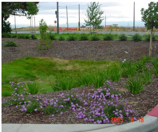
Photo 8-1. Bioretention Area in the City of Fremont
