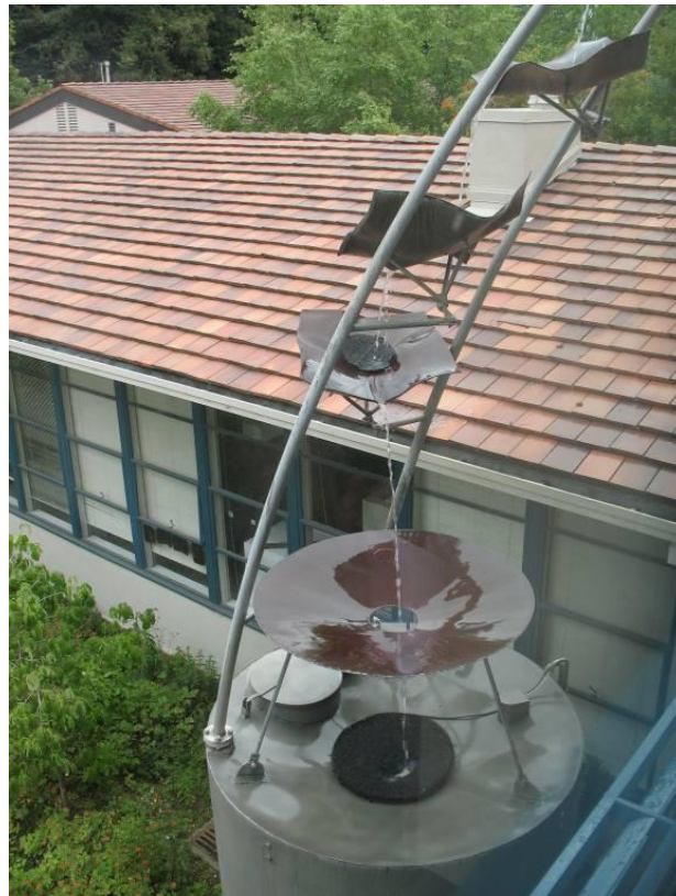
Photo 8-8. Rainwater harvesting system, Mills College, Oakland
